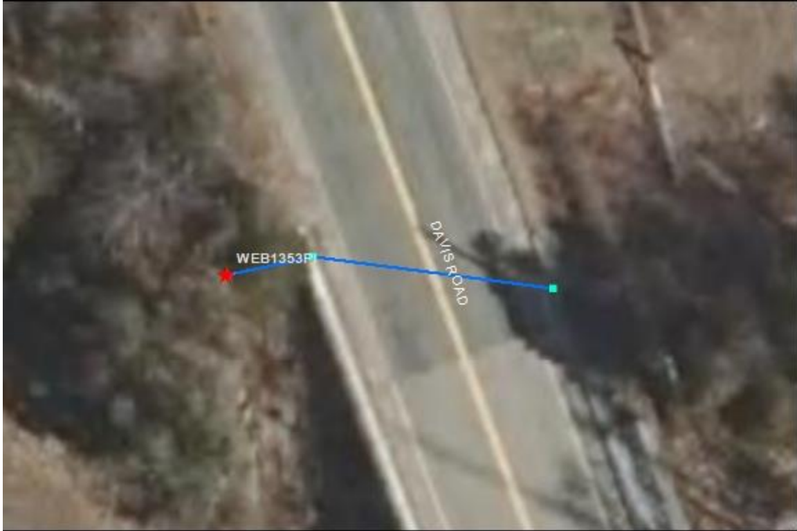
WEB1353PI- Davis Road: No issues found.
