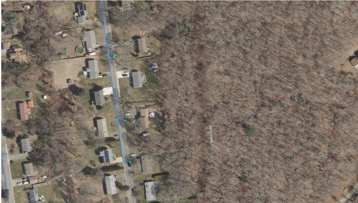
RWP1079PI- Beachwood Drive: No issues found.
