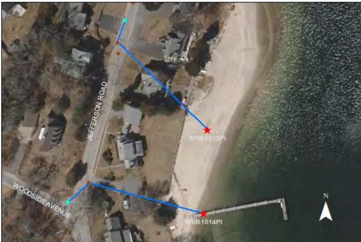
WBB1019PI and WBB1014PI- Jefferson Road: No issues found.
