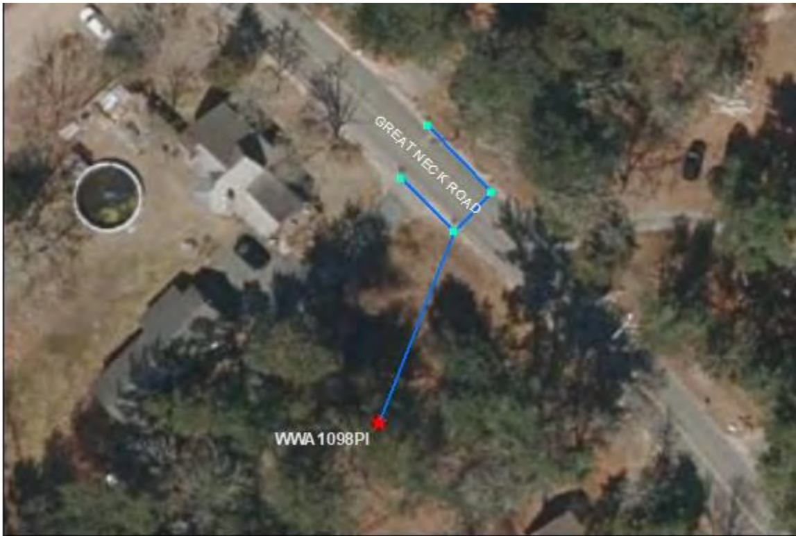
WWA1098PI- Great Neck Road: No significant issues found. There was a strong nature gas odor.
