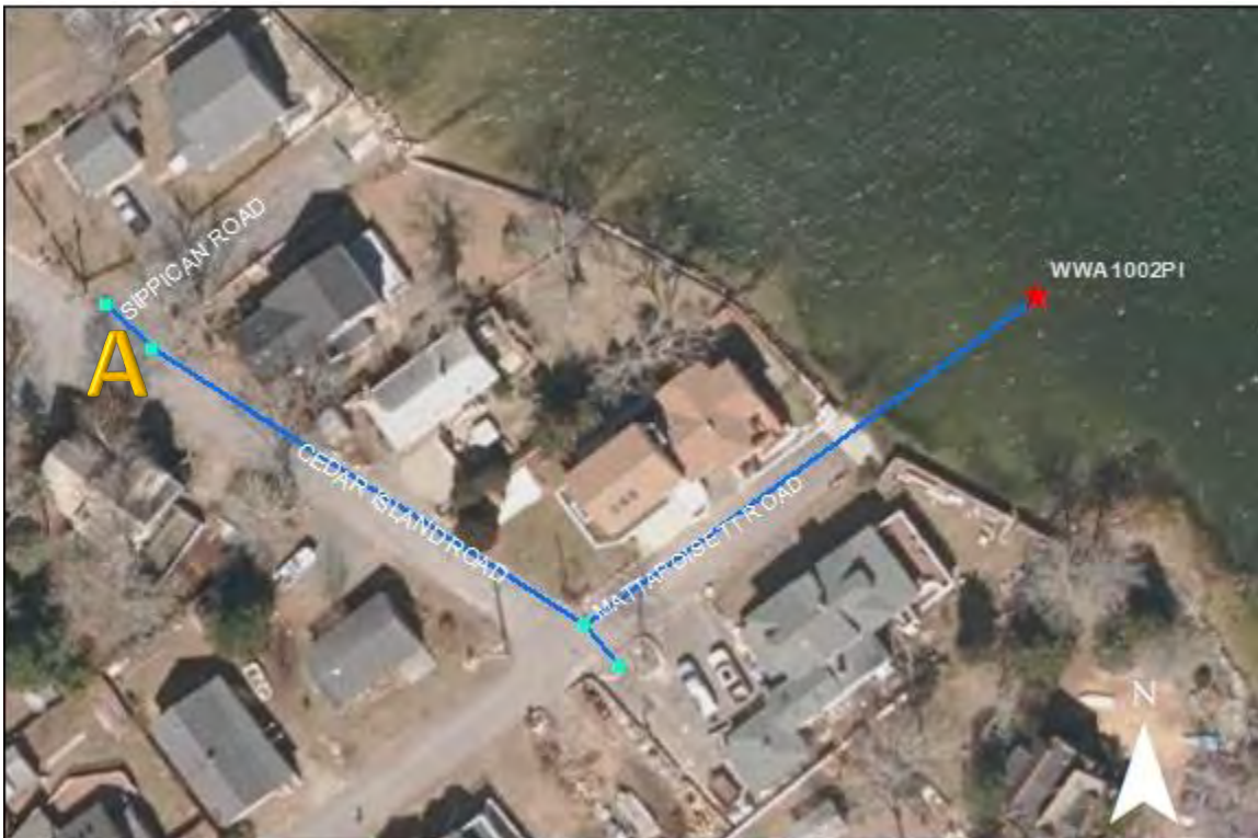
WWA1002PI- Sippican Road, Cedar Island Road, and Mattapoissett Road: At point A there is a very large sink hole. Further attention is necessary.
