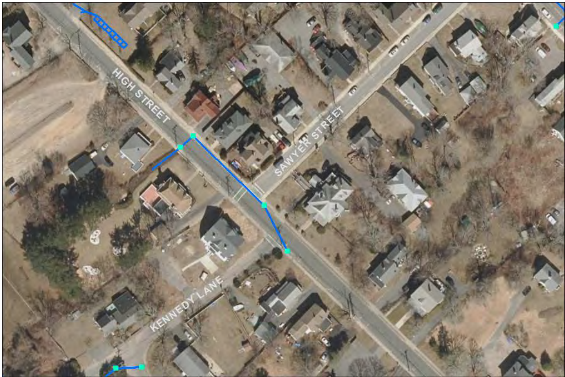
High Street: No issues found; partial network inspection; new asphalt on road – seen observed in structures; this area drains to Broad Marsh.
