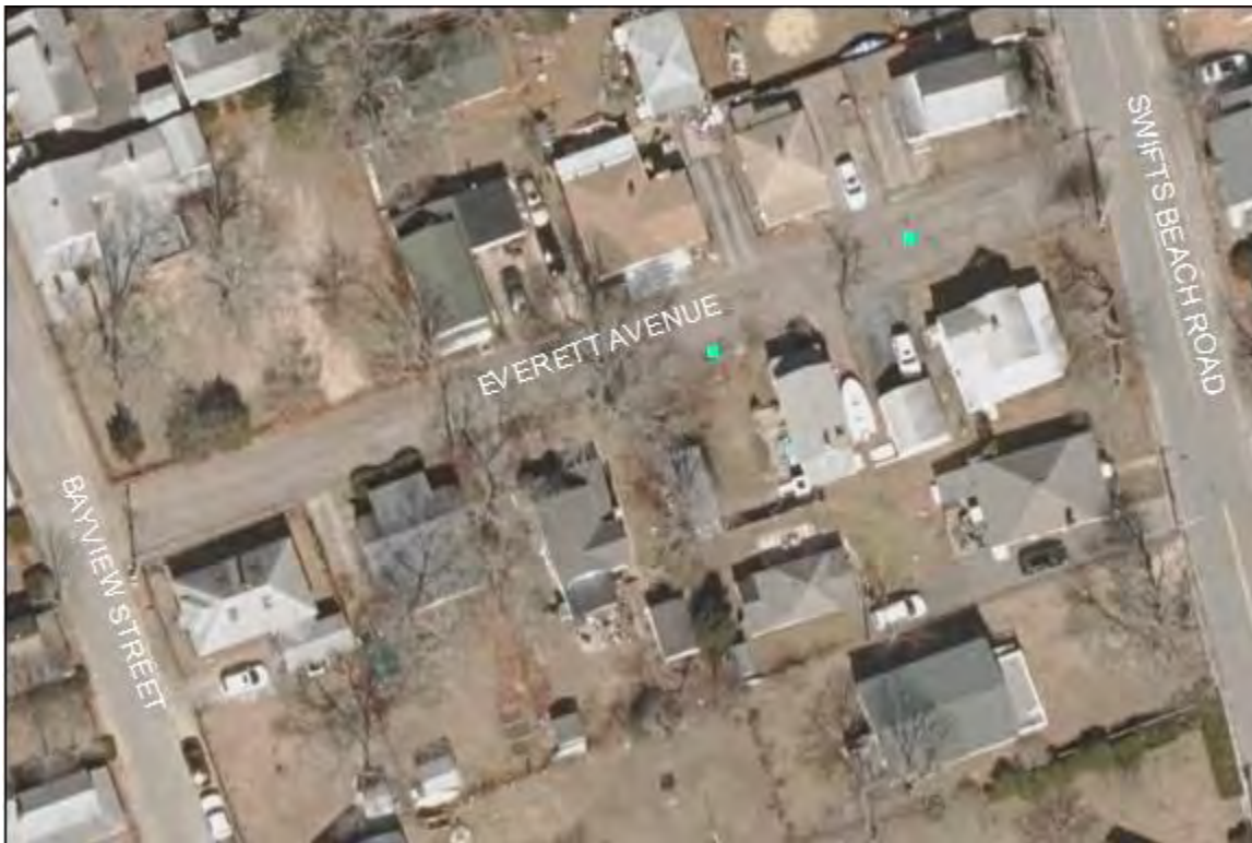
Everett Avenue-. Catchbasins are infiltration basins. The road is dirt and basins are full of sand. Further maintenance is recommended to prevent flooding during rain events.
