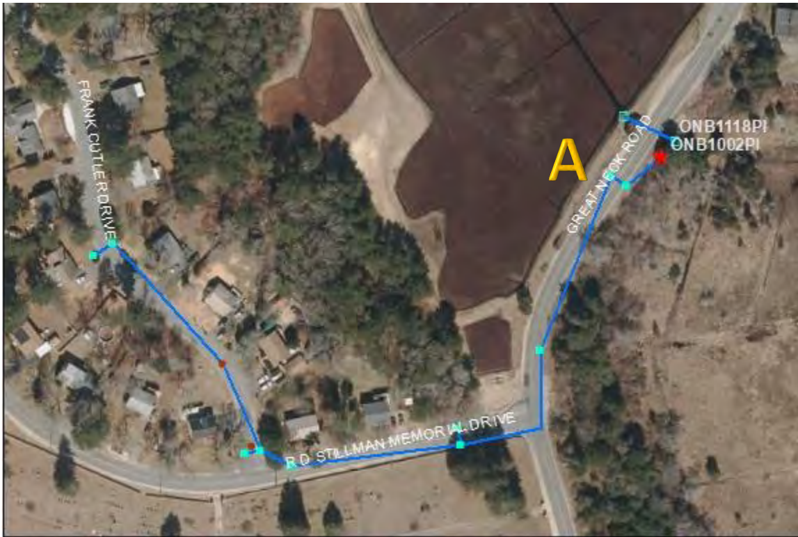
ONB1118PI and ONB1002PI- Great Neck Road: No significant issues found. At point A the catchbasin frame began to sink. Preventative maintenance is suggested.
