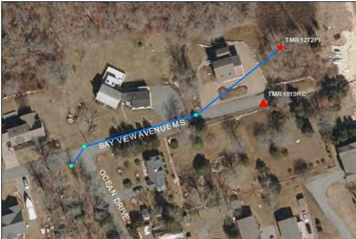
TMR1272PI and TMR1019RC- Bay View Avenue MS: No issues found.
