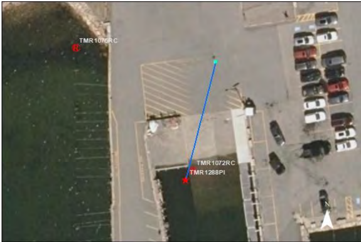
TMR1072RC and TMR1288PI- Marina parking lot: No significant issues found. Suds were observed in the catchbasin. Given that no pipes enter this structure it is likely these suds came from people washing off their boats after pulling them from the water. Educational outreach is recommended.
