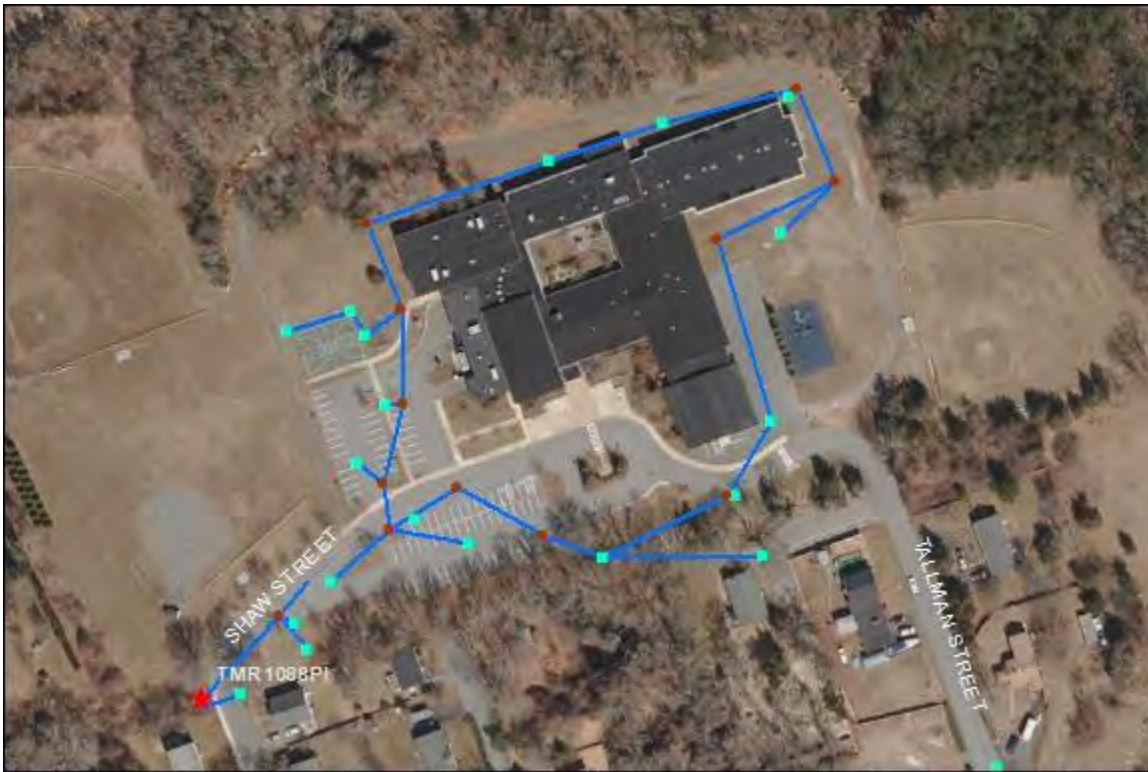
TMR1088PI- Shaw Street at the elementary school: No issues found.
