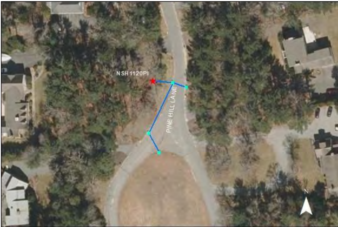
NSH1120PI- Pine Hill Lane: No issues found.
