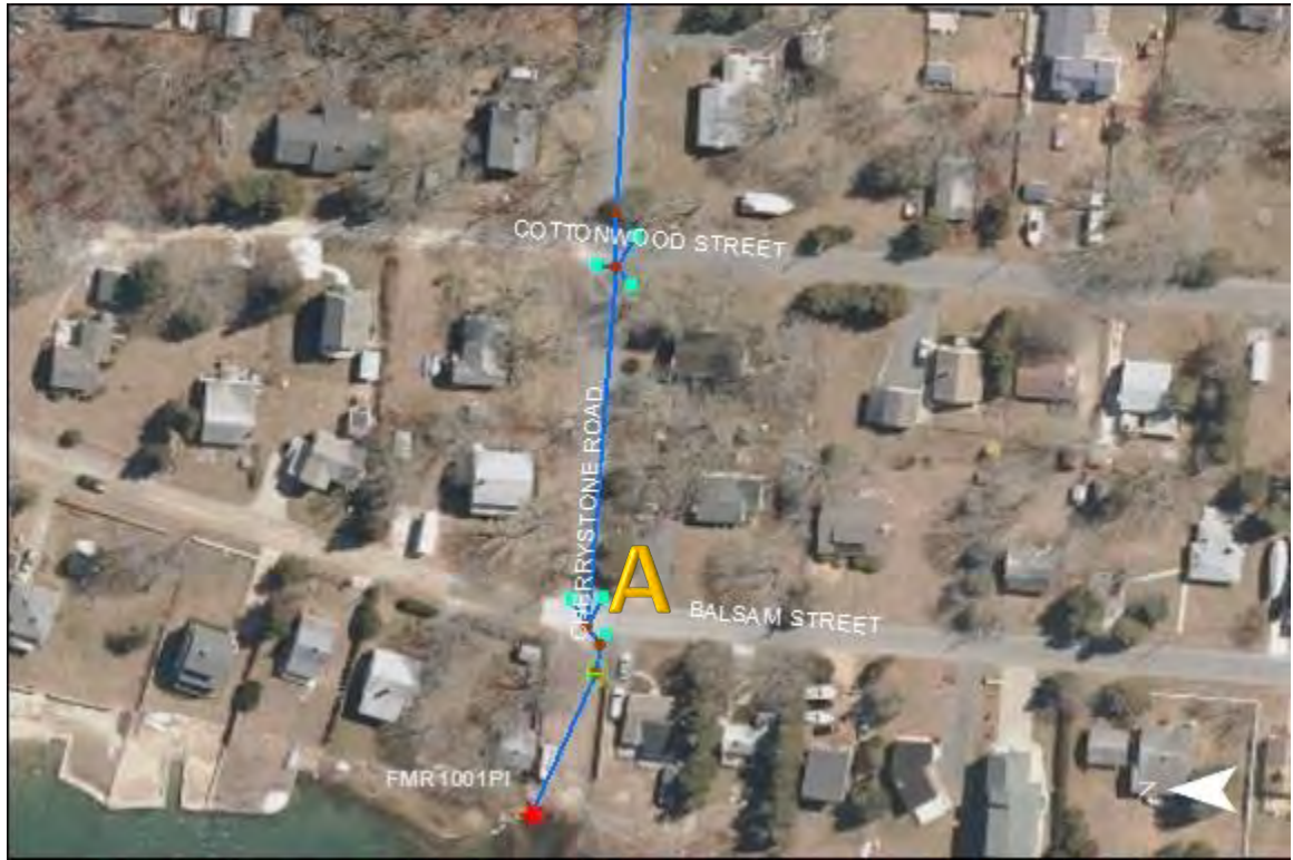
FMR100PI and FMR1001PI- Cherry Stone Road: At point A the catchbasin is sinking. Further maintenance is recommended. Lots of fox excrement was observed in numerous basins and manholes.
