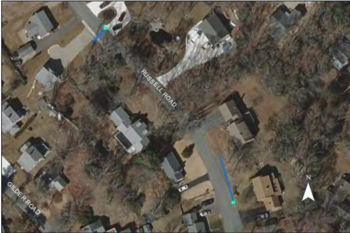
Russell Road: No issues found. The origin of the pipe entering each catchbasin is unknown. Further investigation is recommended.
