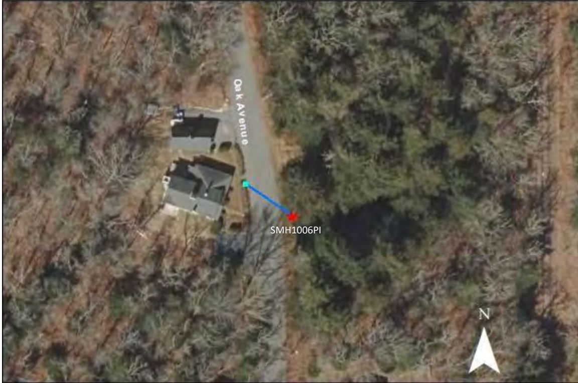
SMH1006PI- Oak Avenue: No issues found. Pipe is buried. Further investigation is suggested.
