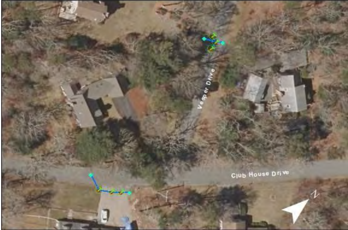
Club House Drive and Vesper Drive: No issues found.
