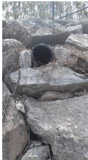
Pipes may be hidden in walls or behind bushes.
