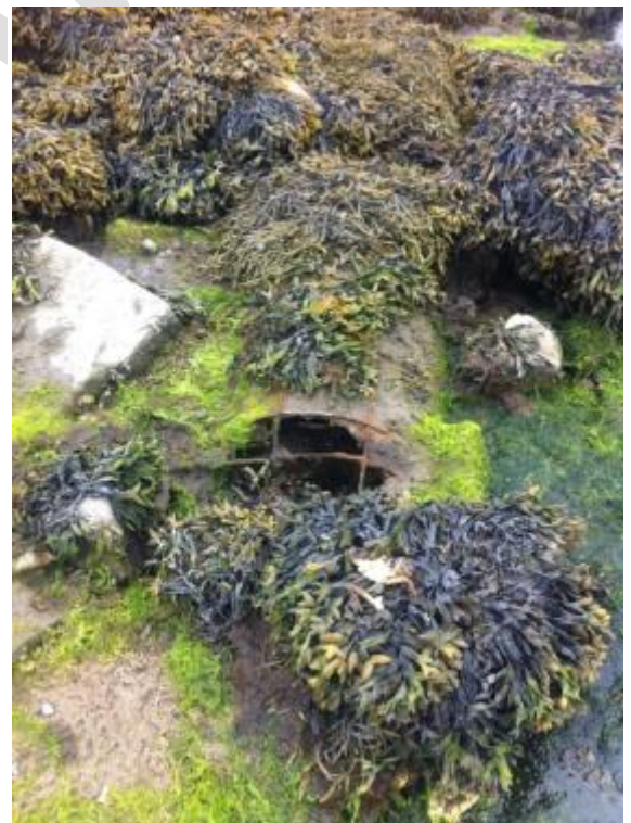
Fig. 7. Many discharges are intertidal or subtidal. Even when they can be sampled at low tide, the sample may be mostly salt water that intruded into the pipe.
